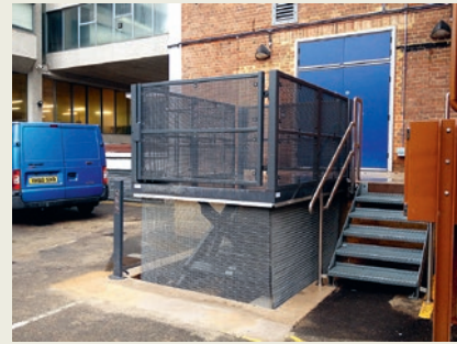
Lorry loader installed in pit, fitted with guard rails, gates and protective wire mesh.
