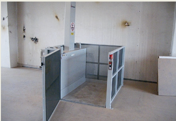
Quick and smooth installation.
