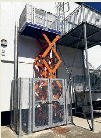
Goods and freight lift
