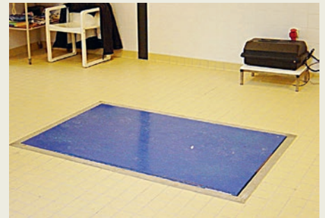
Lift table installed in a pit.
